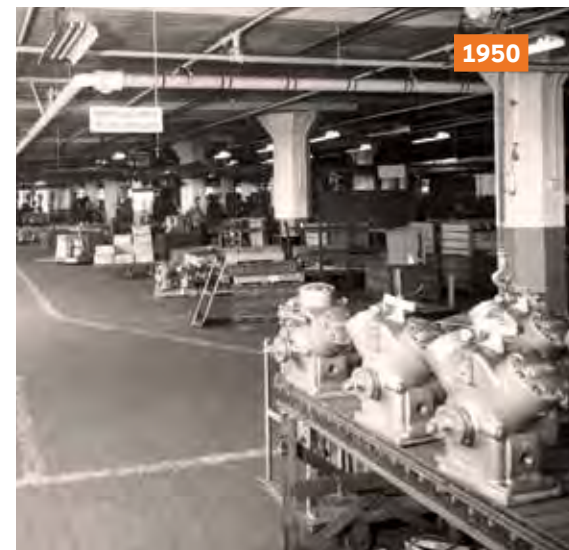
Interior of Carrier’s first factory in Syracuse
