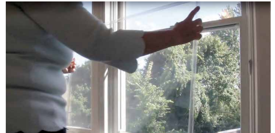
Wex Energy WindowSkin™ is a custom-fit, transparent insulation panel that reduces energy loss when installed on the interior of an existing window for a fraction of the cost of a replacement window.
